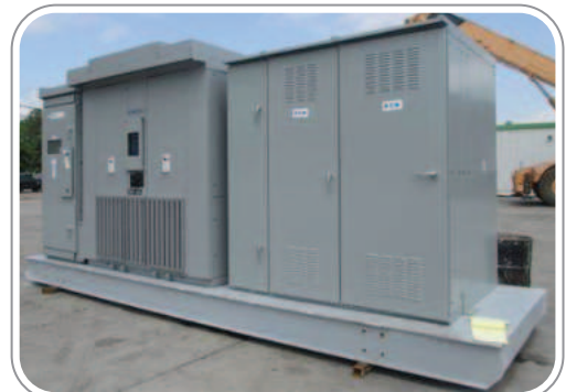
250kV Compact Sub-station (Karnafuli Tunnel)
