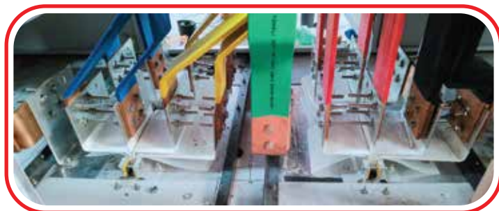
BBT to LT Panel Installation
