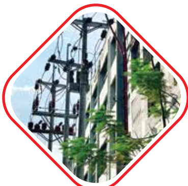
33KV CT,PT & ACR Installation
