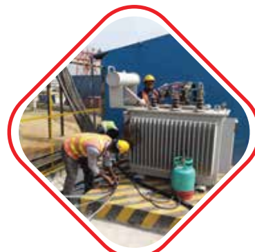
11KV Distribution Transformer Installation
