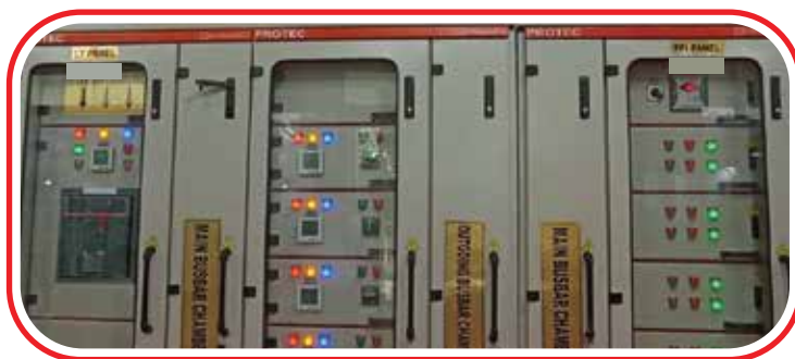
4B Type Motor Control Panel
