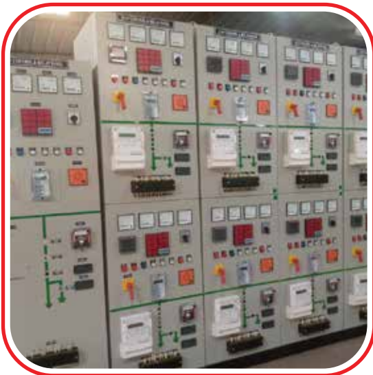
33 KV VCB Control Panel
