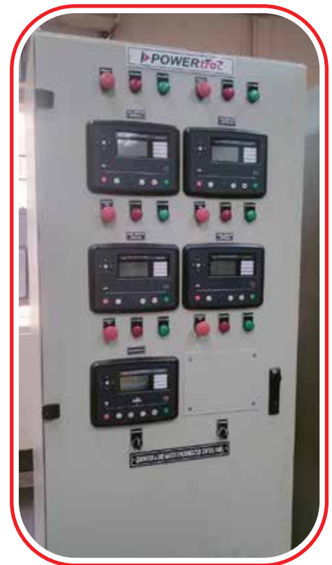
Generator Synchronizing Panel
